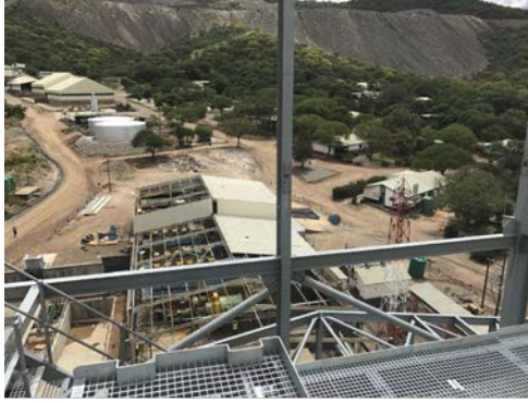
Gecko-Imerys Graphite Processing Facility
